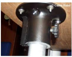
200 lb. man leans on the corner of the table without the pole being fully secured, something had to give. In this case, it was the pole turning in its mounts.
