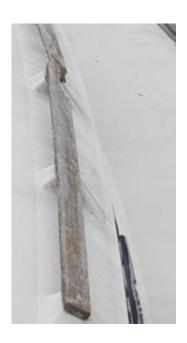
the wood gone, I grabbed the screw and pulled it up as far as it could go so I could cut off the head. Now I figured all I had to do was push the screw back into the cavity until it fell out and then I could fill the holes with epoxy so I could attach the new handrail using Stainless Steel sheet metal screws.
