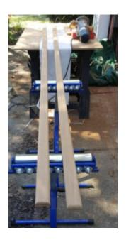
I pre-finished the handrails prior to installation. Once the installation is complete I'll glue in the screw-head bungs using waterproof glue, cut them close to the surface, sand the bungs flush and scuff sand the entire top surface and add some finish to the tops.
